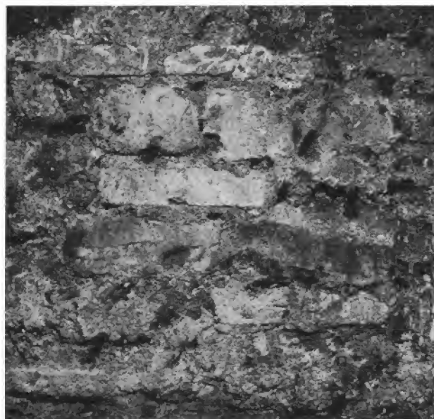
Fig. 170 — S. Marcello al Corso. Opus listatum at the base of the north wall, in the fourth chapel, left (Photo: Sansaini).
